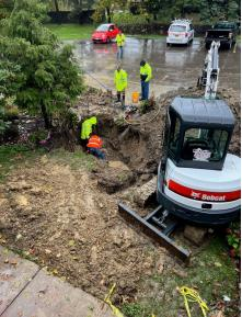
searching. The leak was discovered in an old, undocumented water line that ran under the 400 building and terminated near the waste treatment plant. Thoughts are that the line was installed as a part of the waste treatment plant when the community was still a
